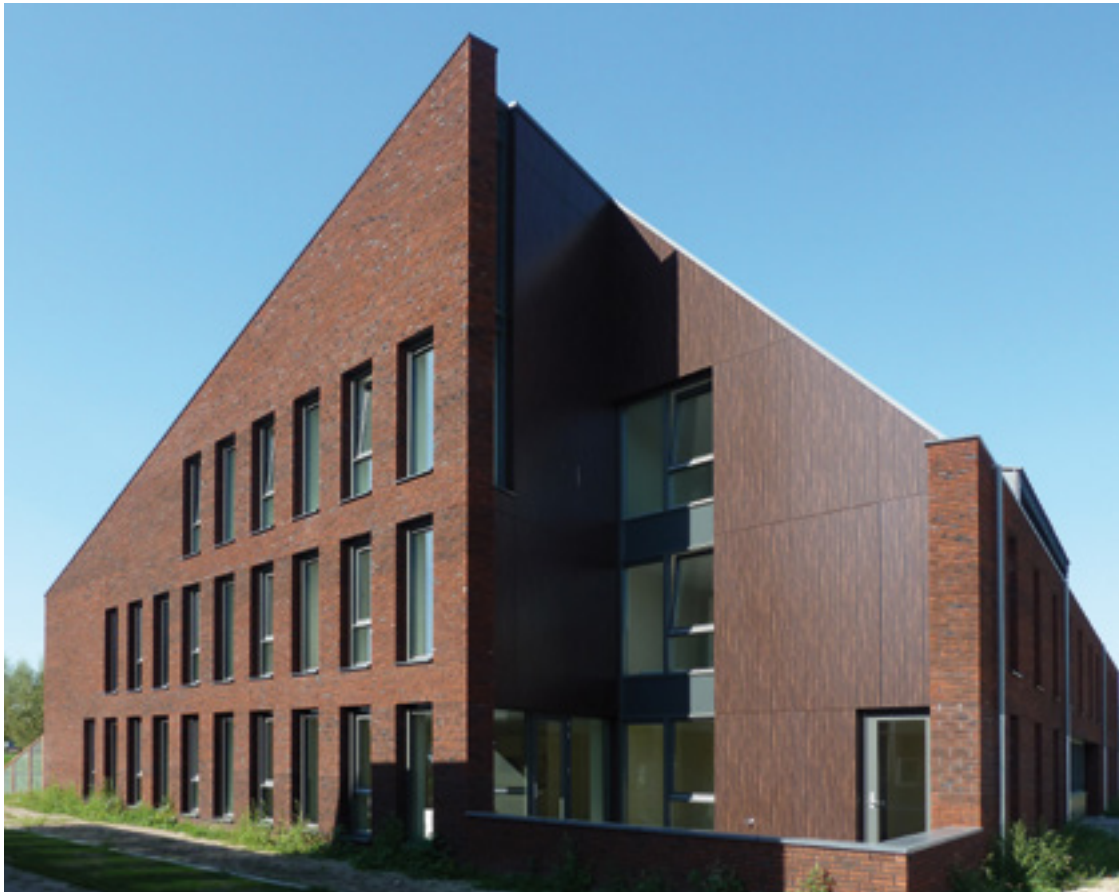
Apartments Beekmos, Houten, Netherlands; Hans Been Architecten BNA, Amerongen, Netherlands
